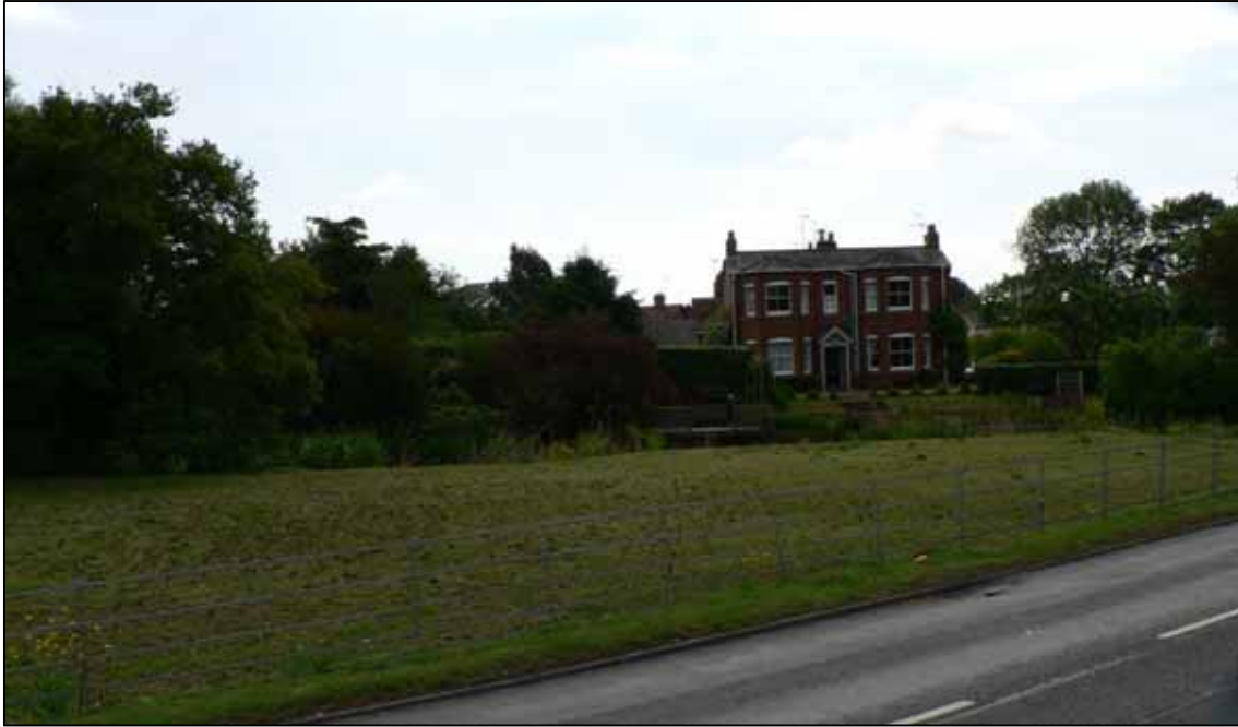
Plate 13: Sightline incorporating the significant view across the Wolston Conservation Area towards the Assessment Site
