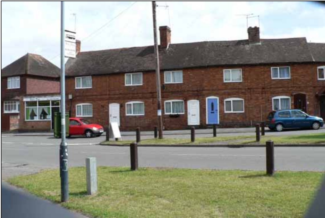
Plate 8: Sightline from the Manor House, Main Street, Wolston (Listed Building 1185673)
